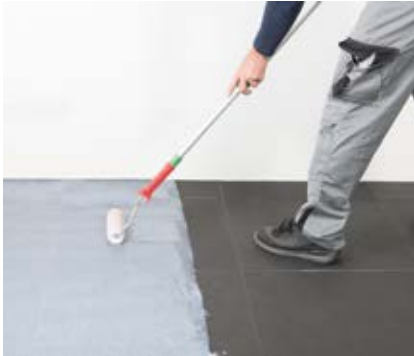
Application of the pressure sensitive adhesive
