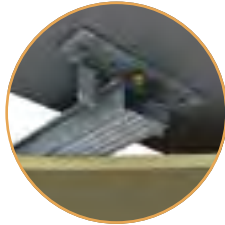
BETAGRIP BG01/02 to Furring Channel NOTE: Centre fixing Only
