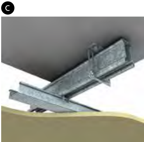
■ INFINITI SLIDING ADJUSTABLE CLIP TO TCR
