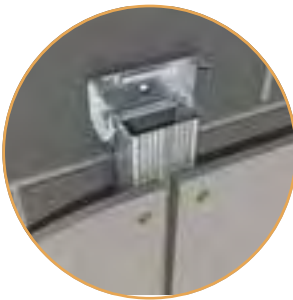
155 Furring Channel Fixed to Wall
